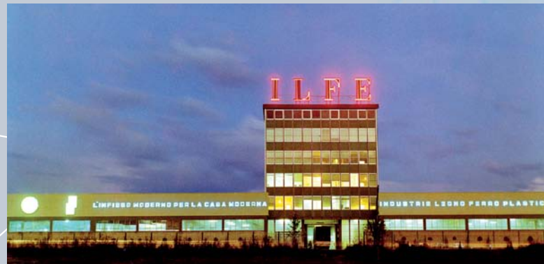
1964: The new factory ILFE Serramenti
