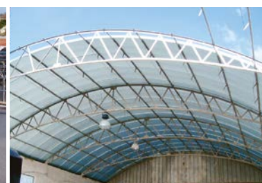
Examples of CURVED ROOF having variable radius and without deflection limitations.
