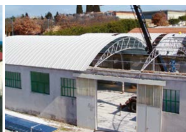
Examples of CURVED ROOF having variable radius and without deflection limitations.
